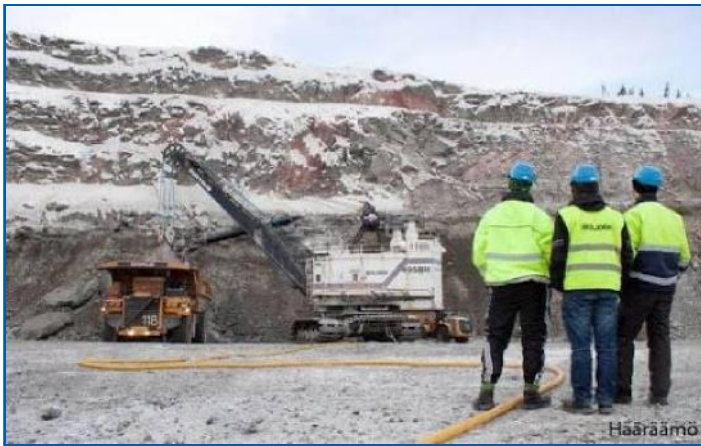
Aitik Mine In Operation During Winter
